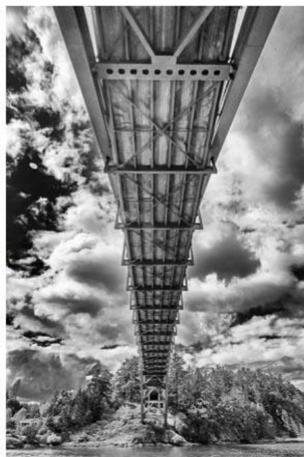
6 Leading Lines Under the Bridge - Sonya Lang
