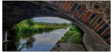
9 Bridge Low Clearance - Renee Deierling
